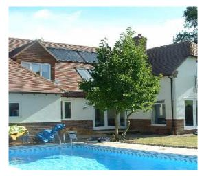
Via a Powertech Thermal Store, this new home in Salisbury also uses the 88 tube solar energy array (two on the east side) to heat the pool once the UFH load is no longer required, at the same time supplying mains pressure hot water on demand
