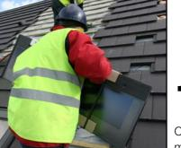
C21 tiles are easily manoeuvred into position on the roof.
