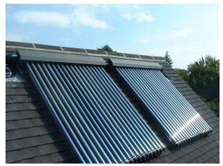
An 88 AP tube heat pipe collector London, UK for part space heating and hot water
